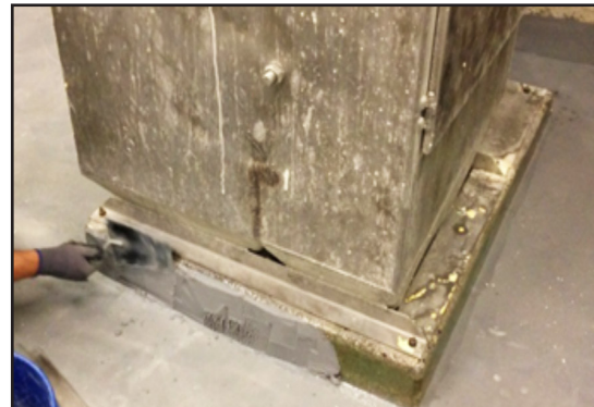
Applying ARC 791 to equipment base
